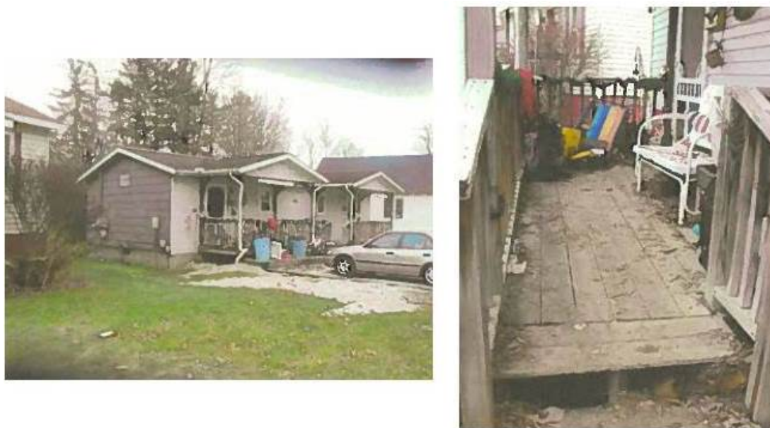
Figure 8. December 2013 Flooded Rental that was recently demolished
