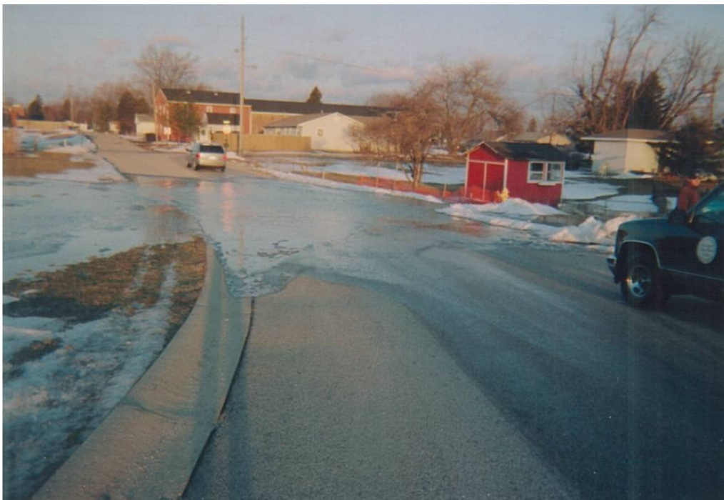
Figure 29. Overtopped Road in Vicinity of Baker Elementary School
