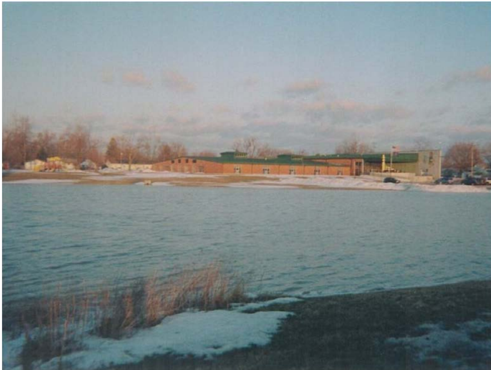
Figure 28. 2008 Flooding a Baker Elementary School
