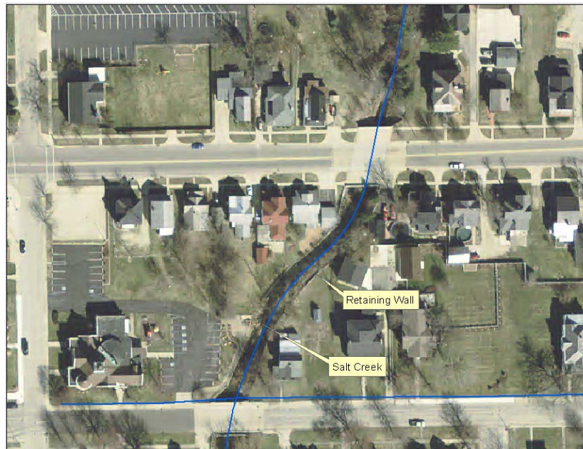
Figure 35. Salt Creek Retaining Walls
